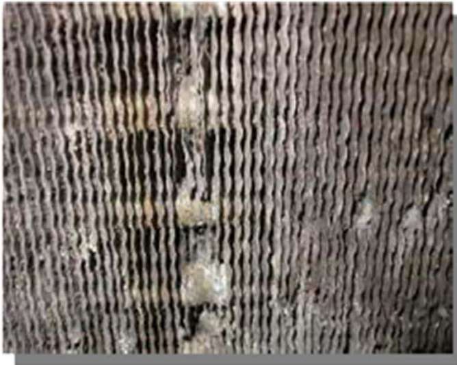
Damaged Coils
