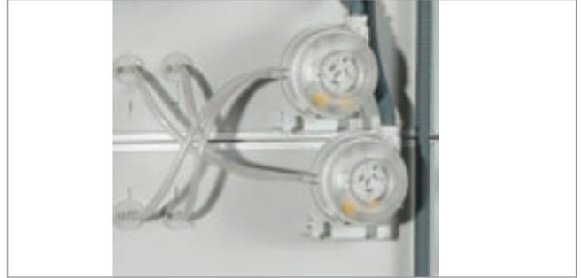
**b) Differential pressure sensor:** It is mainly used to adjust flow rates of the fans and monitor the filter dirtiness in a sensitive way.
